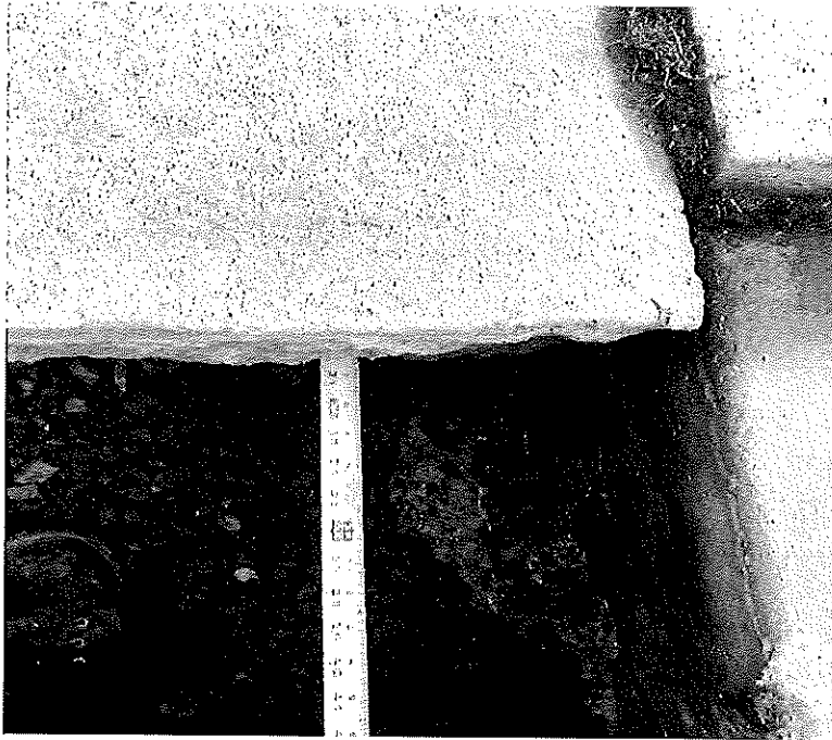
Photograph No. 5 – Measuring tape extending approximately 31 inches east of subsidence area.
