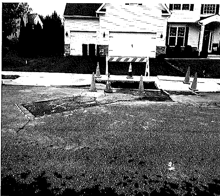
Photograph No. 4 – Previous repair area within Sonoma Way.
