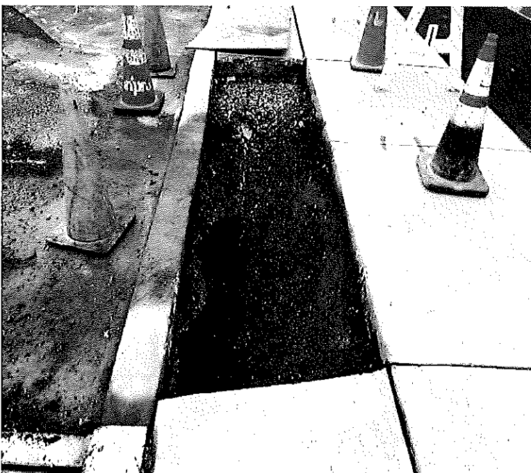
Photograph No. 2 – Area of subsidence within concrete driveway apron looking west.
